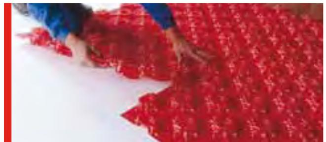
**NOTE:** The 1/2 castellation should overlap the 3/4 castellation. The first panel should be laid with the 1/2 castellation edge against the wall.
