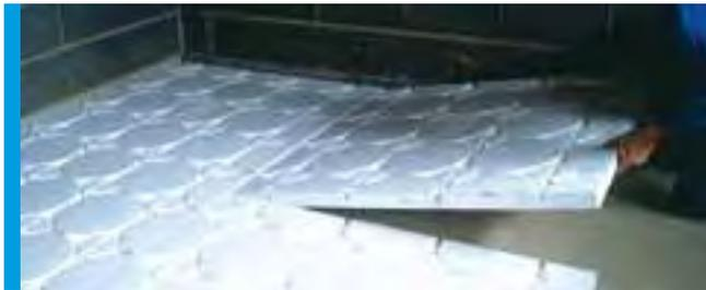
A void in the insulation is often retained around the edge of the room to allow for distribution pipes to be laid from the room to the manifold.
